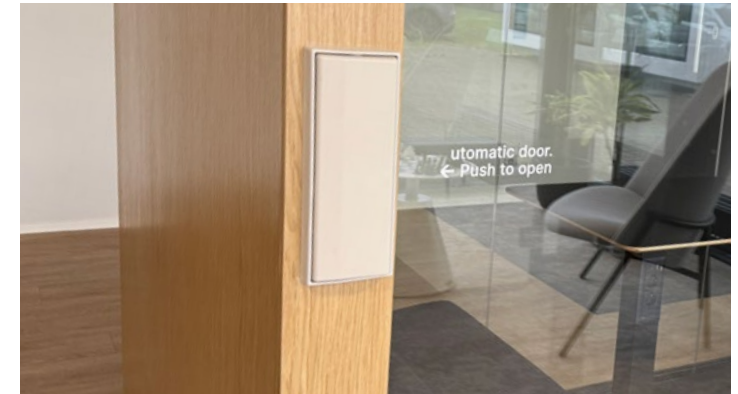
Sensor button for automatic door.
