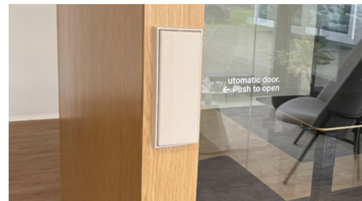
Sensor button for automatic door.
